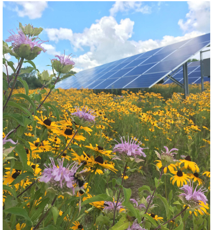
Native vegetation thrives under solar panels. Photo provided by Center for Pollinators in Energy.
